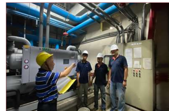
Cooling tower cleaning was conducted, with rigorous supervision of contractor personal protective equipment use and contractor safety training.
